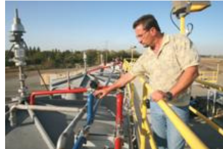
Dave Konwinski, CEO of Onsite Power Systems, shows the pipes on top of the tanks that carry hydrogen and biogases at the Biogas Energy Project at UC Davis. The plant takes food waste and turns it into energy. Greg Rihl/Enterprise photo
