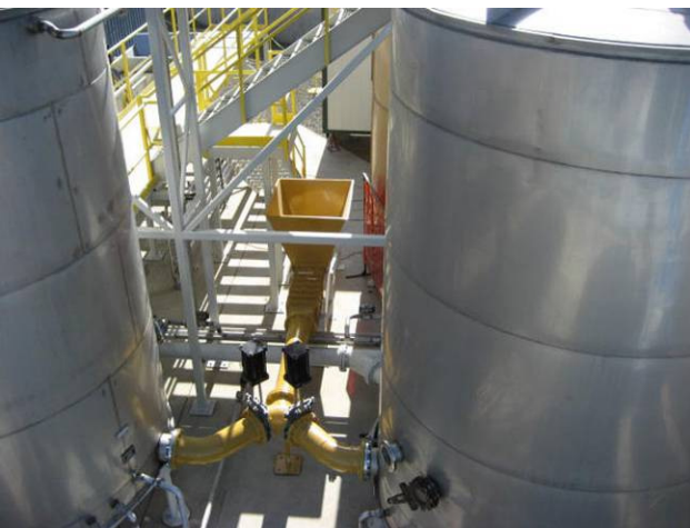
7) The food waste is pumped into the base of the hydrolysis tank through 10-inch pipes. All 8 tons were loaded into the hydrolysis tank in less than two hours.
